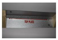
from the left side of the remaining blocks. If the self-tapping screws will not drive past the drywall, stop and try and drive the screw on the other side of the block. It is possible that you have encountered a metal plate protector found over electrical wiring or plumbing.
