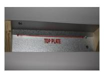
that you have encountered a metal plate protector found over electrical wiring or plumbing.
